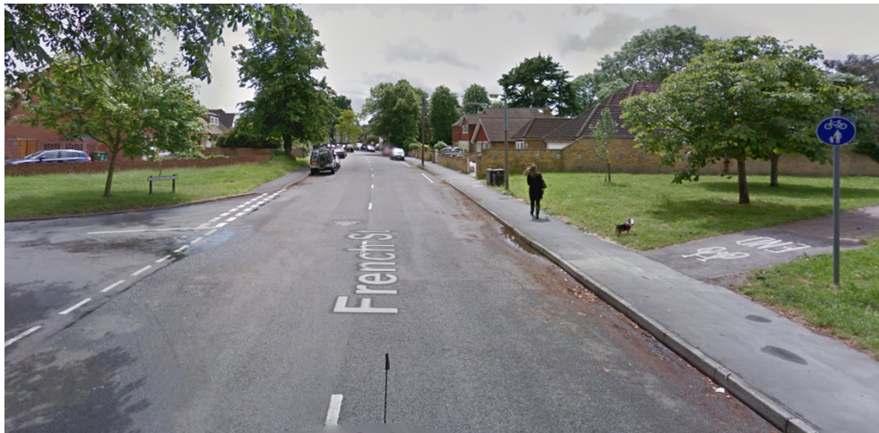
Figure 04: End of Shared footway/cycle way on French Street
