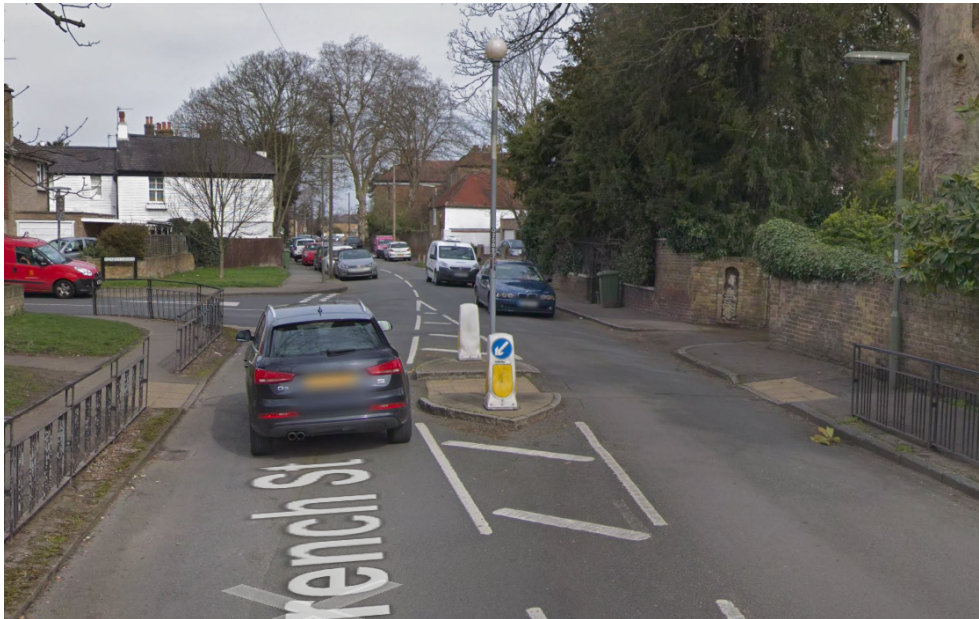
Figure 02: Pedestrian refuge island and on street parking within the current 20mph zone.
